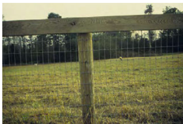
Figure 5. A top rail added to a square mesh fence prevents horses from stretching the fence wires. An electric fence wire installed on the opposite side of the post will prevent horses from rubbing on or chewing the board.
