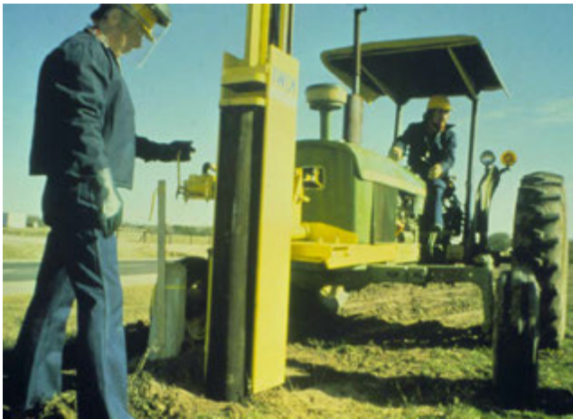
Figure 11. A tractor-mounted post driver.
