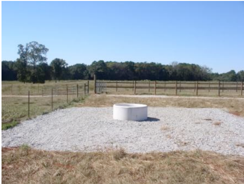
Figure 2: Prefabricated Concrete Watering Tank on Heavy Use Area
