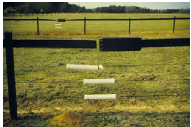
Figure 2. A high-tensile fence with top “rail.” Tensioning devices are covered to protect horses from cuts and to allow the fence to be “dropped” quickly if a horse becomes entangled.
